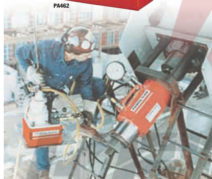
PA554 pump and RH2008 Center Hole cylinder used to tension cables.
